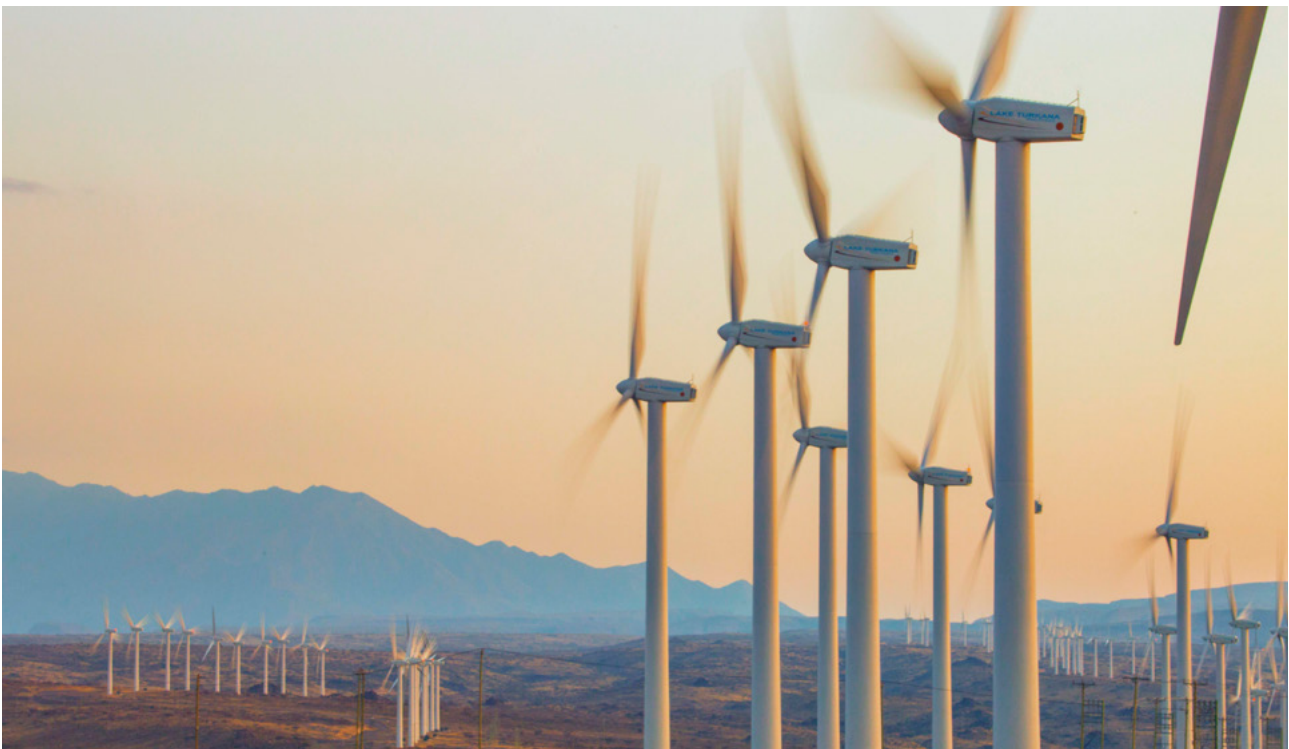
In 2018, Africa's largest wind farm Lake Turkana Wind Power was connected to the national grid. Finnfund has been a shareholder in the company ever since the construction began in 2013.
