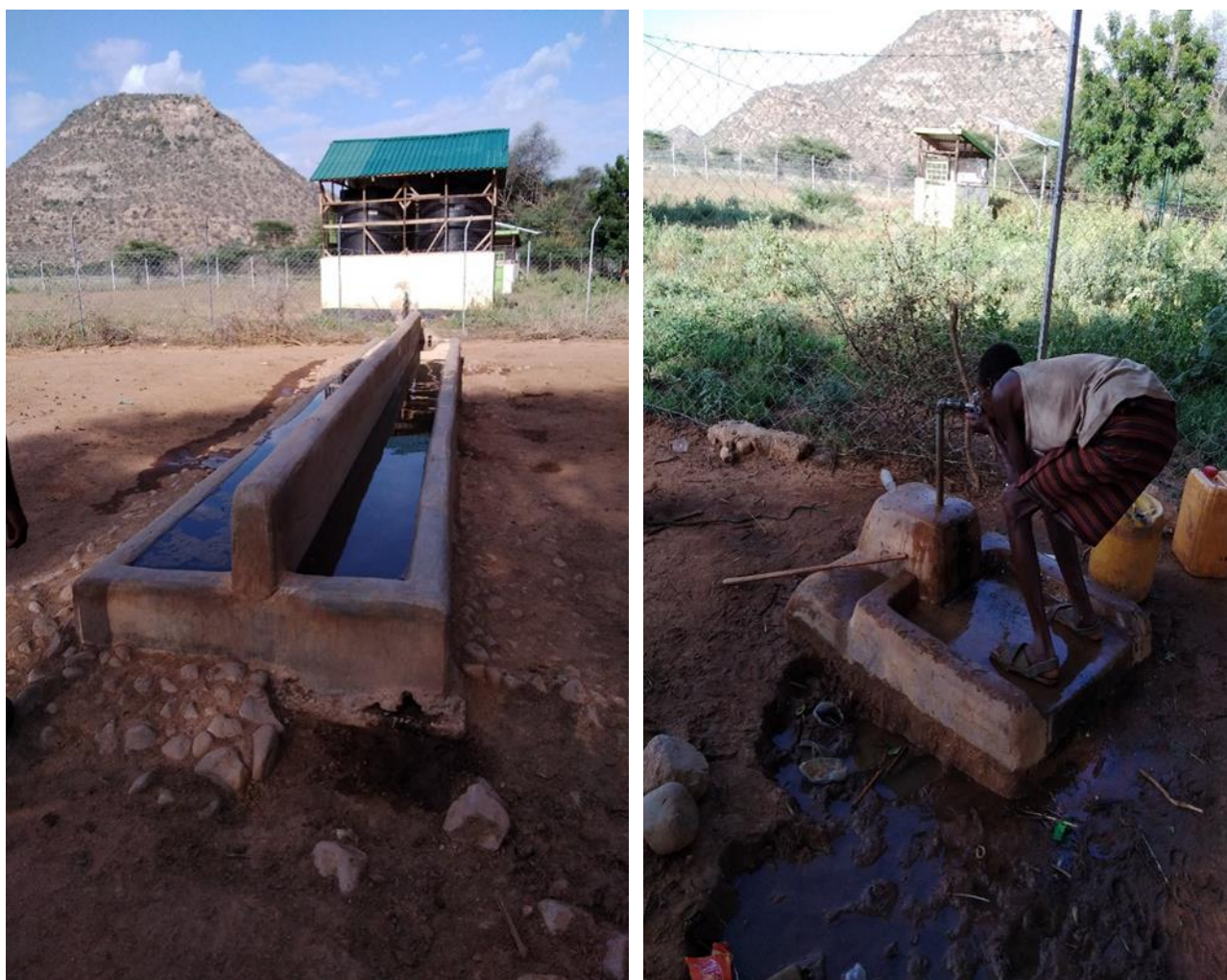
Figure 6.4: Borehole drilled by LTWP in Ntil village
